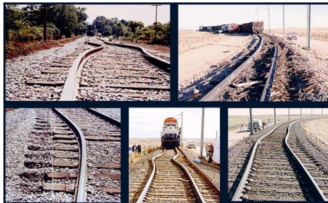
FIGURE 6.21 – Flambement de rail.
