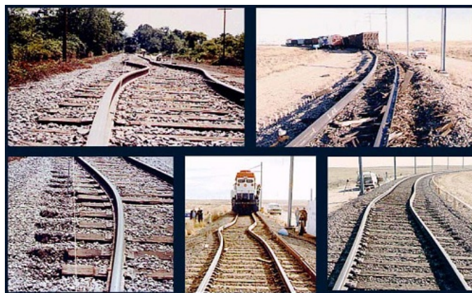
Figure 6.21: Rail bucking.
